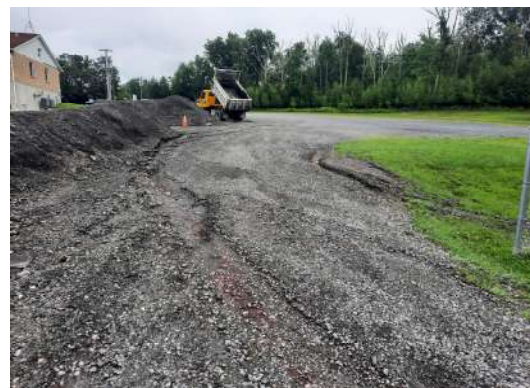
DPW yard pinches entrance to field
