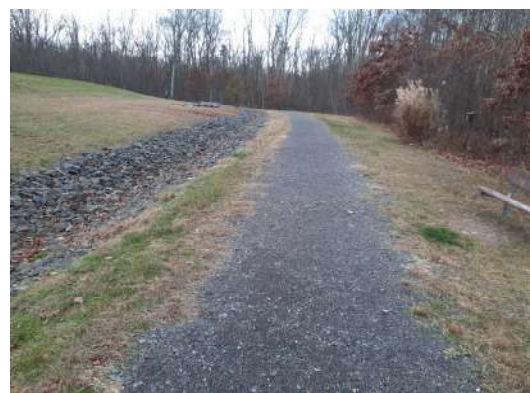
Trail system with drainage swales
