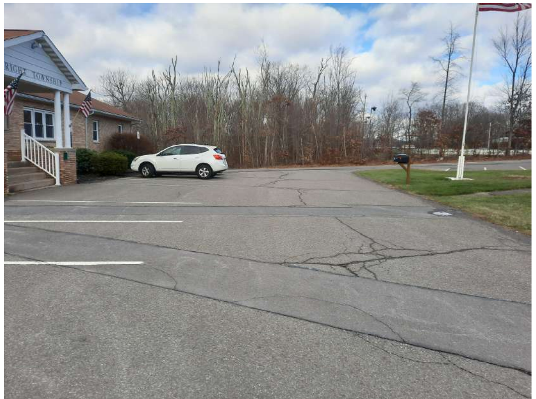
Municipal Building Entrance & Parking
