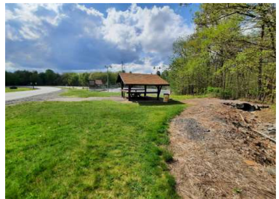
Kiwanis shelter along Park Road
